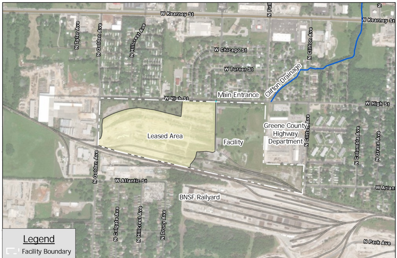
The former Tronox/Kerr-McGee Wood Treatment Facility in Springfield, Missouri, is outlined in white.
