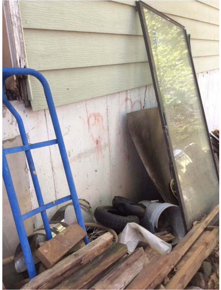
Cracks in the poured concrete shown from the west side of the exterior.
