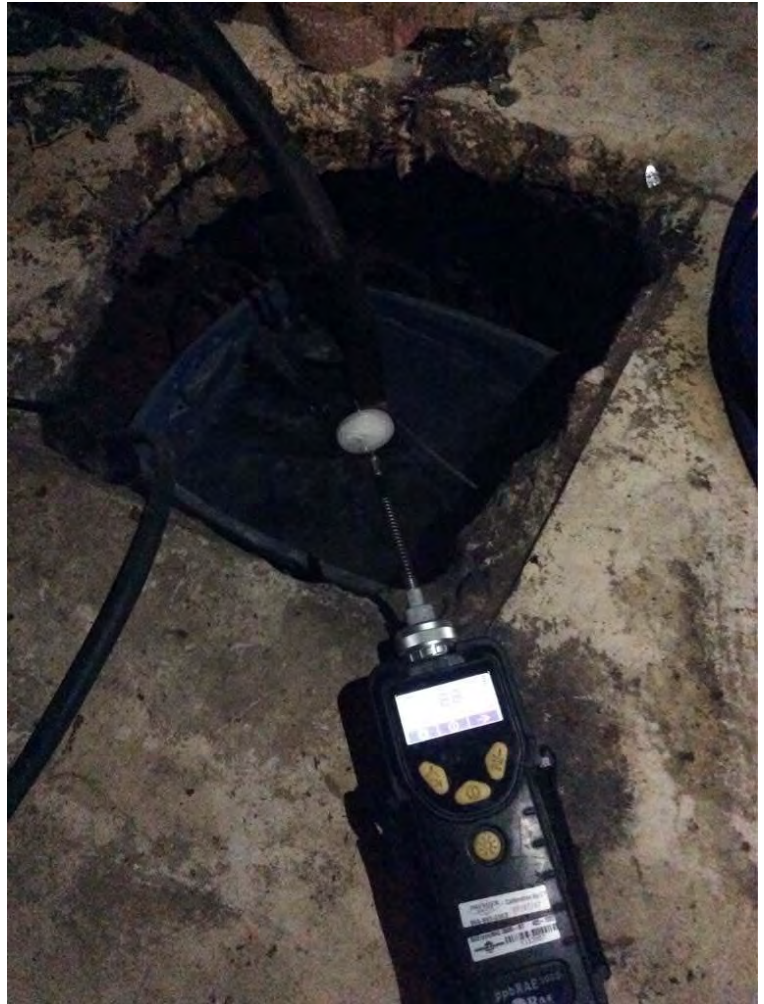
Sump located in the north corner of the basement.
