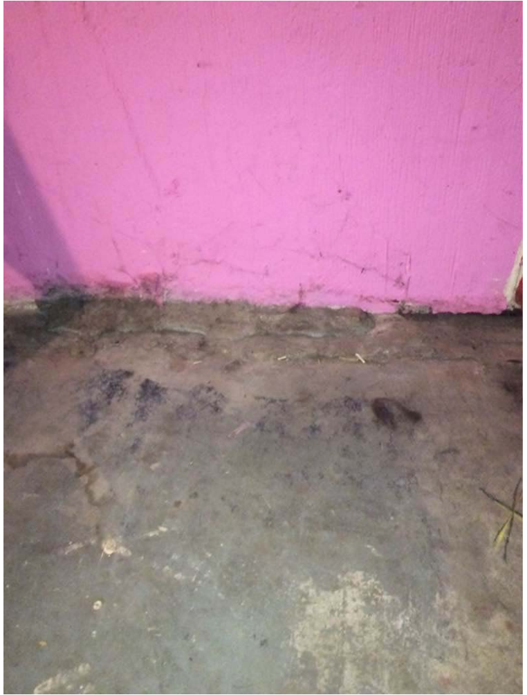
Crack between exterior south side wall and floor appears to have been filled at some point.
