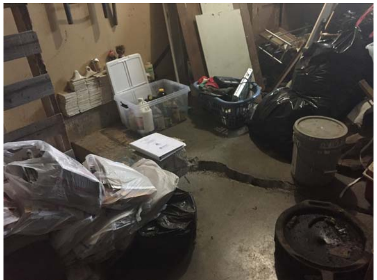
Crack between exterior south side wall and floor appears to have been filled at some point.
