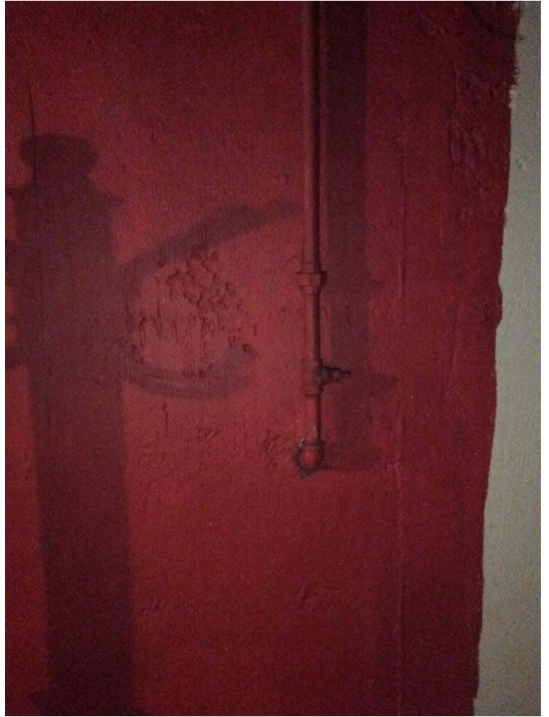
Water line along south side wall.
