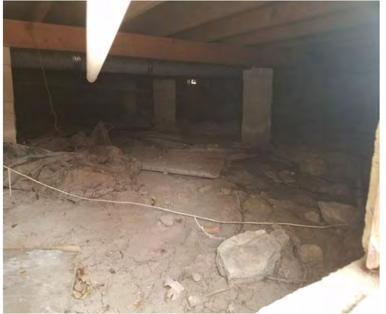
Crawlspace, looking southeast. Far side vent is uncovered.
